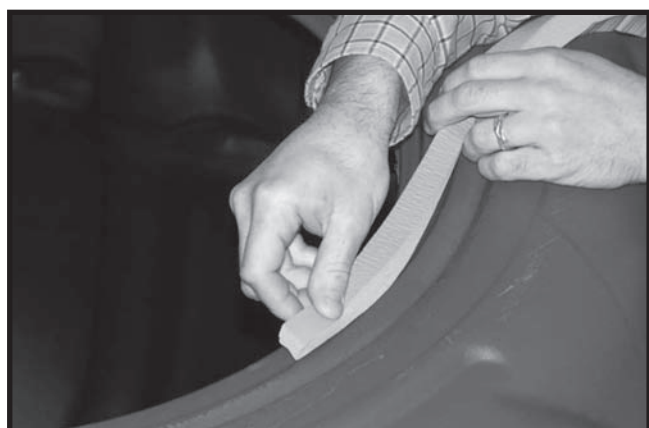
FIG.2 Apply Gasket
